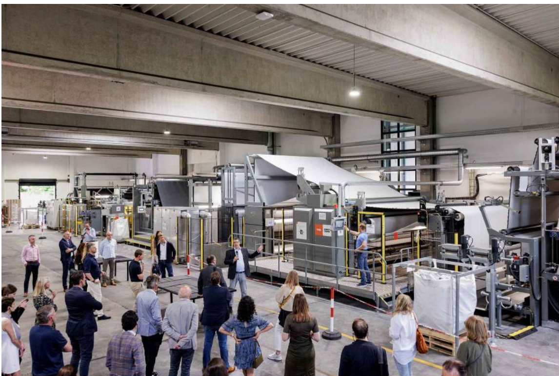
A novel coating system where the process requires no gas or water and uses up to 95% less energy than conventional production methods Photo: Simon Wegener
